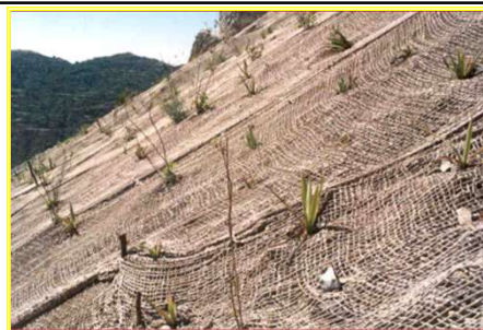
Geojute matting for slope stabilization
