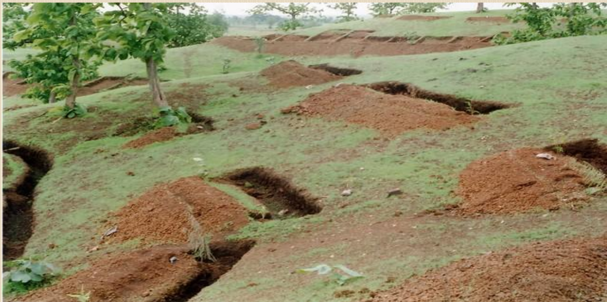
Staggered Contour trenches
