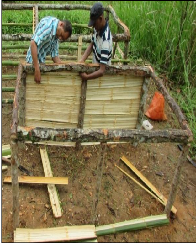
Fig 1: Construction of enclosure unit
