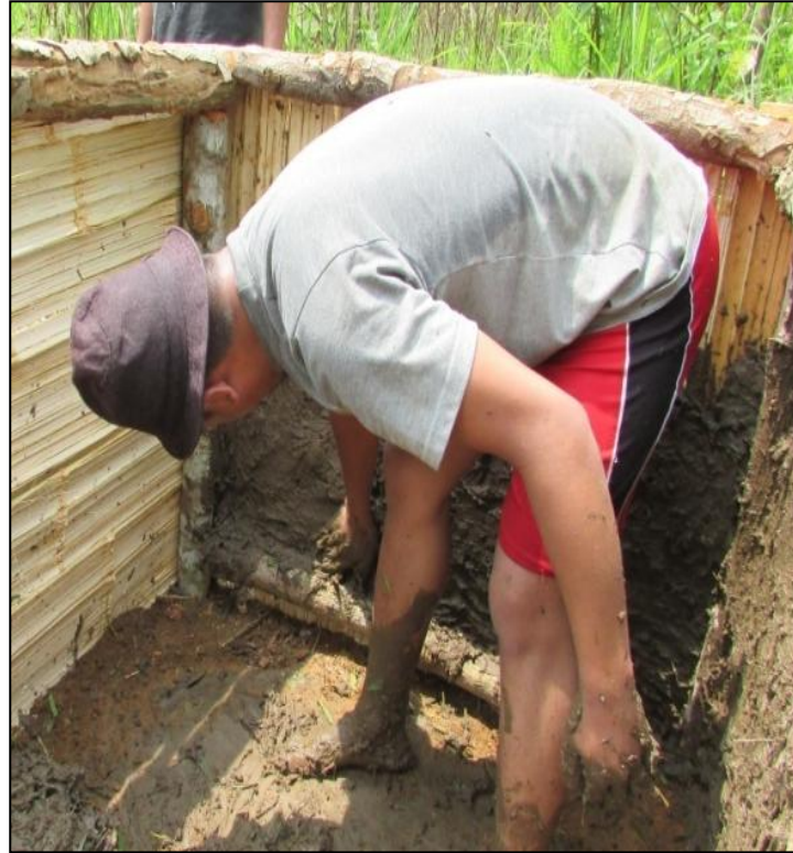
Fig 2: Plastering of the compost floor and walls
